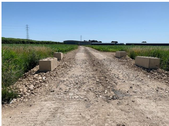
Photograph 13 New temporary road through the arable land.
